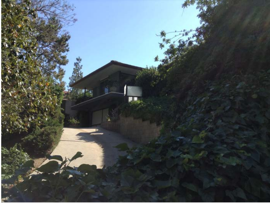
The deep eaves and corner overhang of this 1962 Ranch house are suggestive of a Japanese influence. It has an original stack bond retaining wall (property 31).
